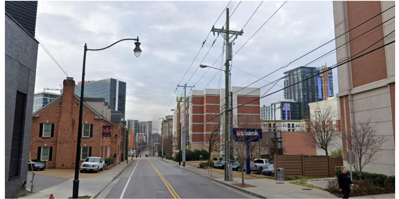
DIVISION ST - LOOKING WEST
