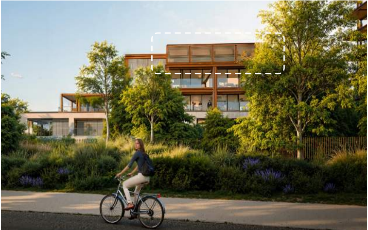
AHU TYPICAL SCREENING
